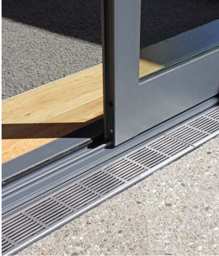
1. the threshold must allow for wheelchair access
