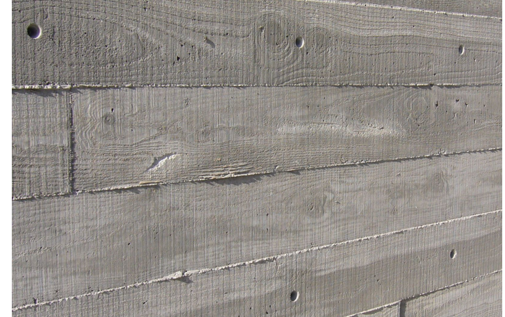
5. concrete made using timber formwork
